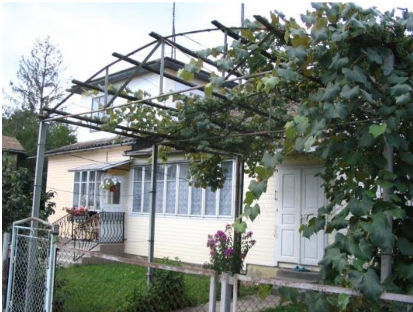
Solotwin, general view
